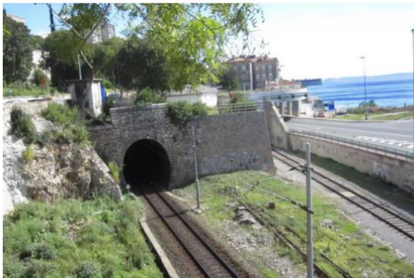
Fig. 1. Tunnel Brajdica before reconstruction.
